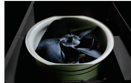
Newly designed curved air discharge bell mouth for better aerodynamics.
