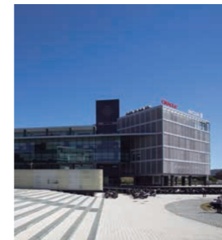
Andalucia Technology Park. Málaga, Spain. ECOi
