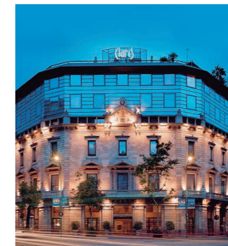
Hotel refurbishment. The heat recovery system is ideal for a hotel of this category. Hotel Claris 5*. Barcelona, Spain. ECOi
